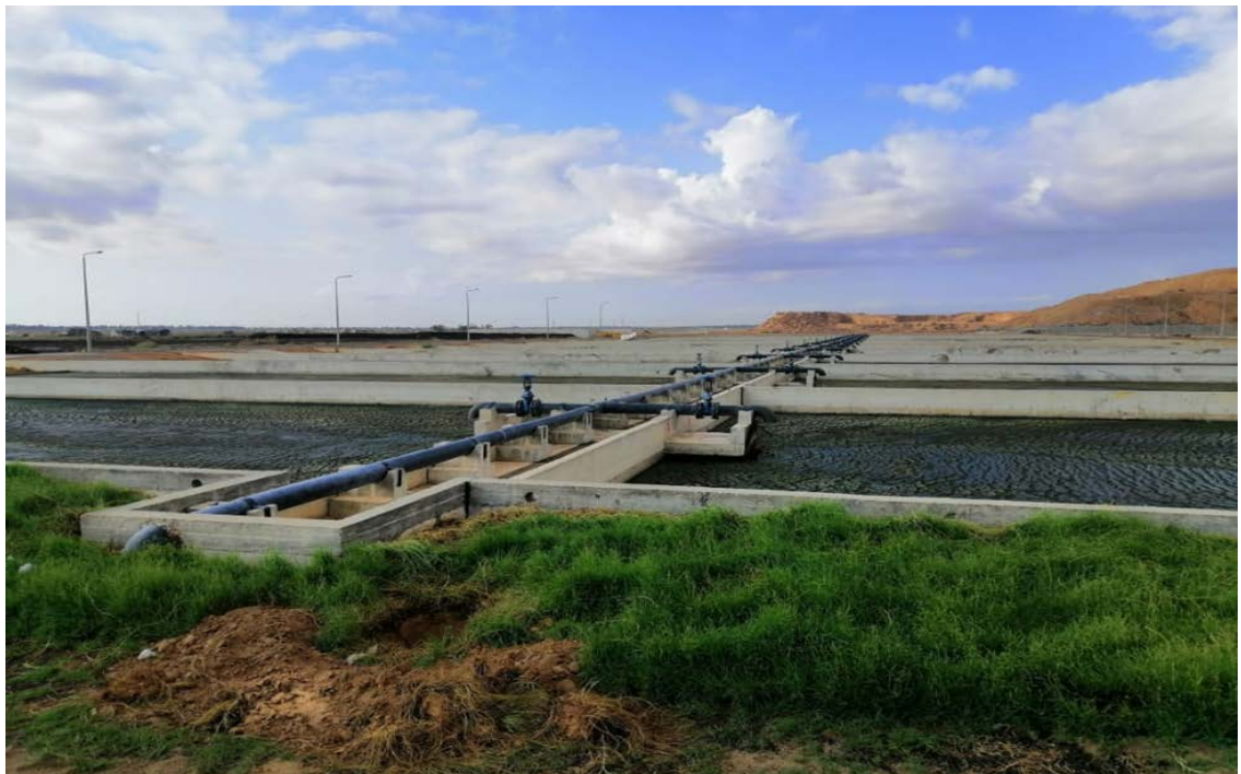
Sand Filter Under Operation up to June 2020
