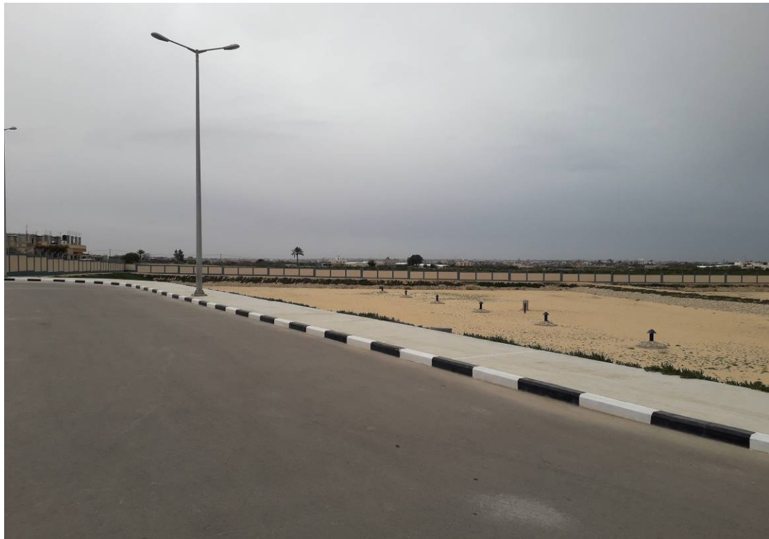
Boundary Wall for the Infiltration Basins up to Completion in January 2020
