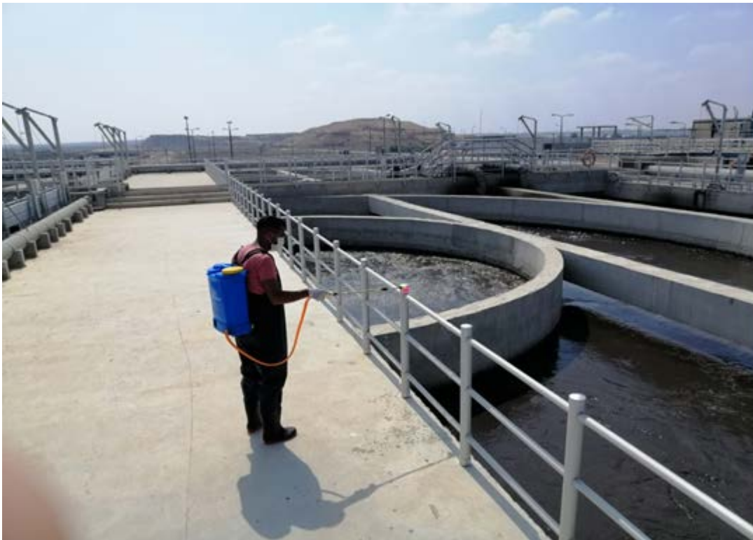
Disinfection measures in KY WWTP against COVID-19
